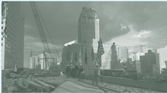
DEBRIS ON ROOFTOPS NEAR WORLD TRADE CENTER (COURTESY OF FEMA PHOTO LIBRARY)
