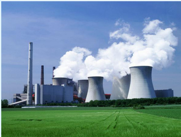
A COAL-FIRED POWER PLANT (COURTESY OF WIKIMEDIA COMMONS)
